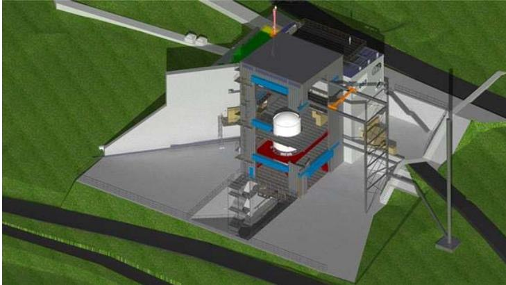
What it will look like – the test rig P5.2. The upper stage of the Ariane 6 will be tested extensively on this new test rig at the DLR site in Lampoldshausen. These include fuelling and defuelling tests and hot running tests for the upper stage. The commissioning is scheduled to begin in 2018.
